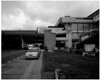
West view with relics of ramps and passages, 2008
